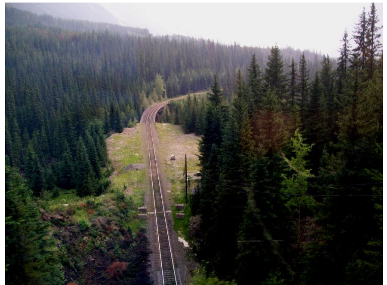
(Right) Exiting the Upper Spiral Tunnel at Kicking Horse Pass
